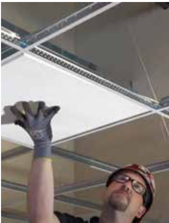
1 Place Precut Panel Into Grid 1" Cutting + Waste Eliminated
