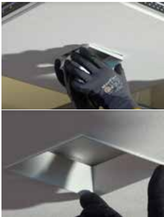
3 Insert USAI's Trimless Acoustical Trim
