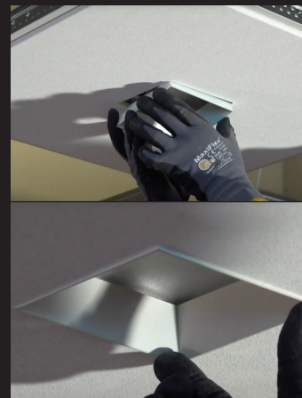
3 Insert USAI's Trimless Acoustical Trim
