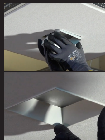
3 Insert USAI's Trimless Acoustical Trim
